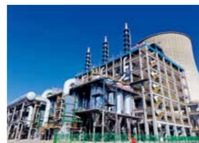
新疆宜化 3×40000 m 3 /h 循环流化床气化炉 3 units of 40000 m 3 /h CFB Gasifier in Xinjiang Province
