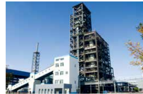
甘肃金化千吨级加压循环流化床气化炉 Pressurized CFB Gasifier with the Capacity of Kiloton/day Grade in Gansu Province
