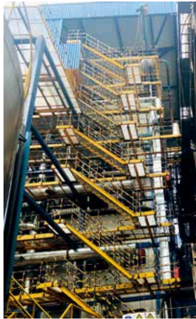
山东邹城 40 吨 / 时煤粉预热燃烧锅炉 40 t/h Preheating Pulverized Coal Combustion Boiler in Shandong Province
